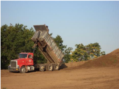
Perimeter Flood Protection – stockpile of top soil
