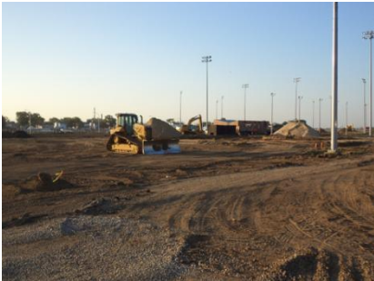
Perimeter Flood Protection – East Park Reconstruction
