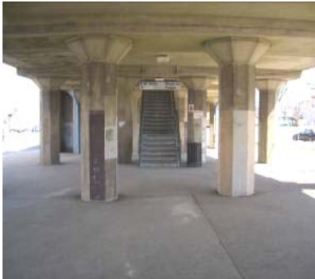
One of the staircases leading up to the platform
