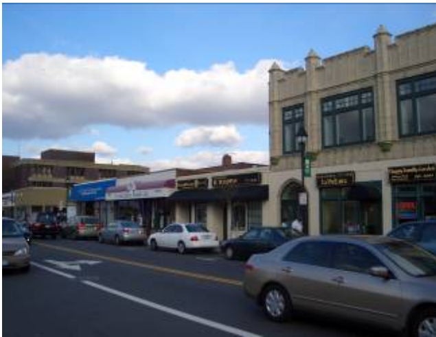
One- and two-story commercial buildings
