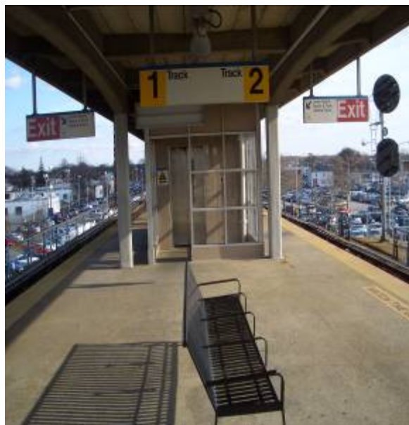
View of the elevator from the platform level
