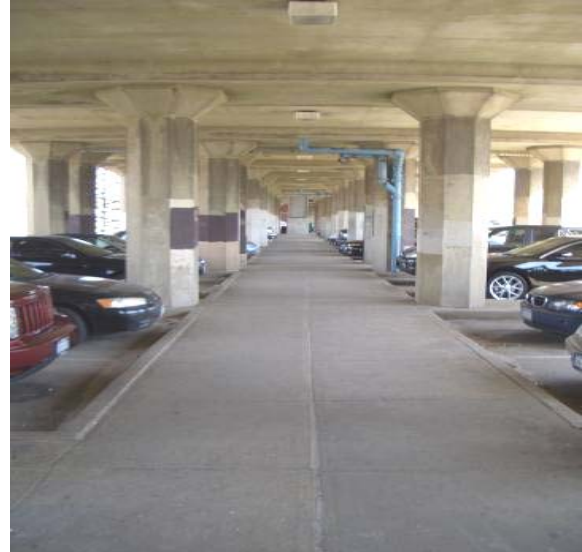
View along the pedestrian underpass
