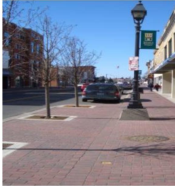
Brick pavers and planting strips
