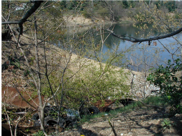
Figure 8 - This storm water recharge basin (SWB), also known as a sump, holds water all year long. These basins sometimes become a dumping ground for old tires and debris, which can collect water and serve as ancillary breeding sites for mosquitoes. NCDPW tries to remove these items on a regular basis.
