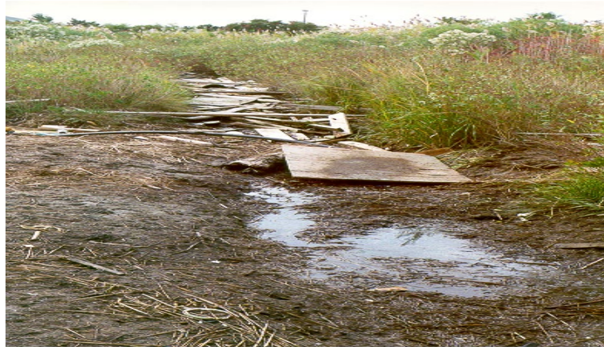
Figure 10- This floodwater ditch, filled with sand and debris, is in need of maintenance to prevent mosquito breeding
