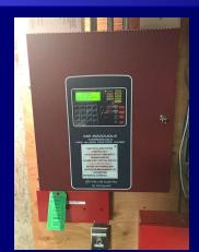
The fire alarm control panel is the brains of the fire alarm system the control panel interprets signals from initiating devices activates notification devices and may control doors fans or many other building systems the control panel should be checked daily to ensure that it indicates normal operations in the event that the control panel indicates any trouble or supervisory conditions this should immediately be reported to the appropriate party to ensure correction
