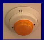
The initiating devices of a fire alarm system are devices such as pull stations, smoke detectors, heat detectors, and Carbon monoxide detectors that initiate activation of the fire alarm system. Pull stations should be located adjacent to all exit doors and should be checked daily to ensure that they are not obstructed by displays objects or any other items. Smoke, Heat, and Carbon monoxide detectors should not be capped or covered.
