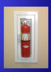
When checking the portable fire extinguishers look for the following. Have the portable fire extinguishers been inspected within the last year, do the gauges show the proper pressure, is it the correct type extinguisher for the area served and Is it mounted and clearly visible
