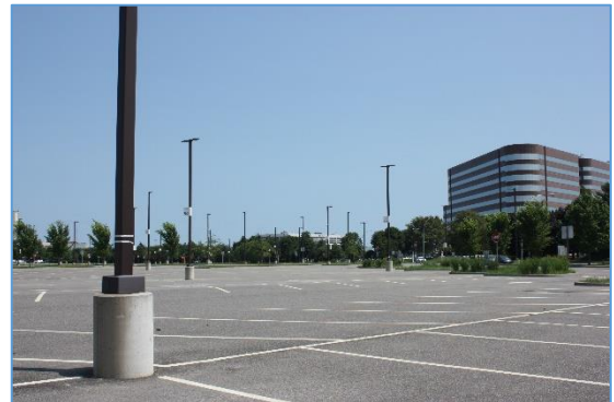
2: View looking southeast towards the subject property from Museum Row. The Omni building is visible on the right.
