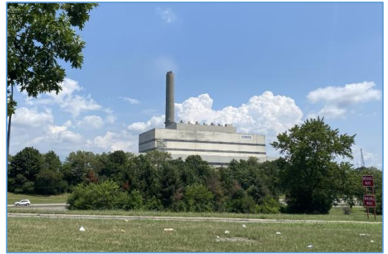
5: View looking west towards the Reworld™ Hempstead Facility from Merchants Concourse.
