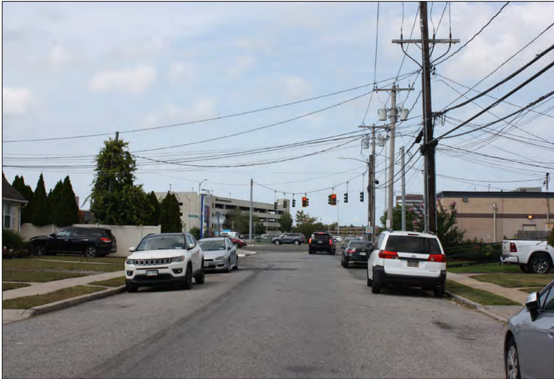
Existing Viewpoint 12: Intersection of Hempstead Turnpike and Cunningham Avenue
