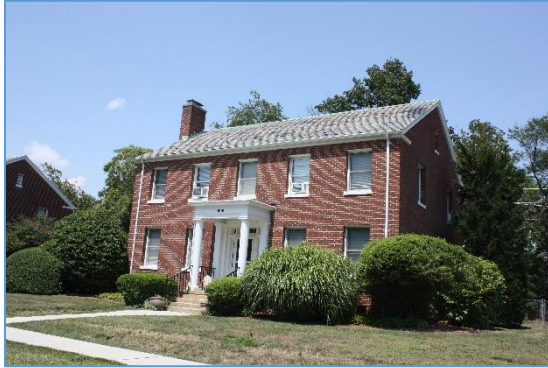
3: View looking west towards the NCO Housing on Bane Road within the Mitchel Air Base and Flight Line Historic District.
