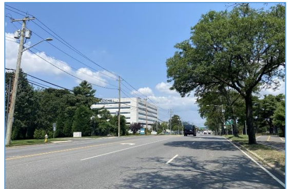
14: View looking north on Merrick Avenue towards 425 Merrick Avenue, west of Eisenhower Park.
