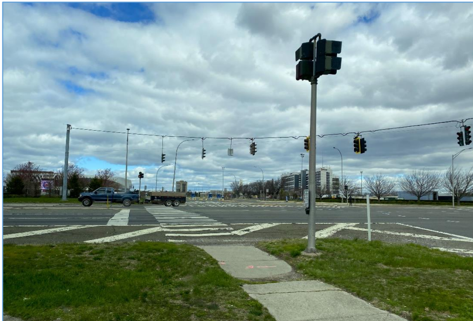
Photo 11: View from Hempstead Turnpike and the intersection of Glenn Curtiss Boulevard looking north towards the subject property. The Marriott Hotel is visible toward the right of the photograph, with the Nassau Community College Administration Building located at a distance at center of the photograph.
