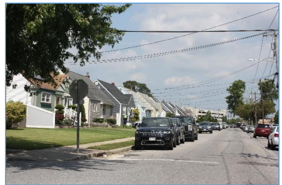
9: View looking north on Cunningham Avenue towards the single-family residential homes south of Hempstead Turnpike.
