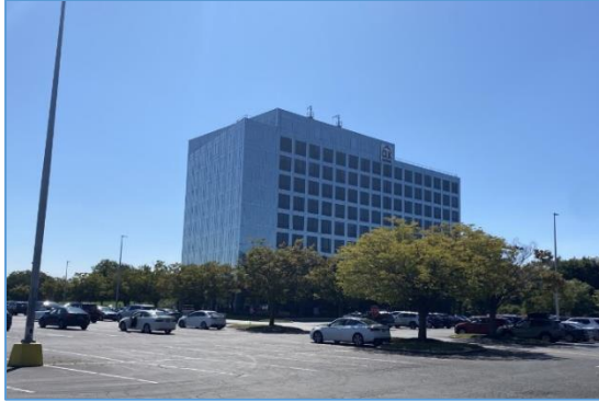
6: View looking southwest towards the 90 Merrick Avenue office building from the northeast corner of the parking lot.
