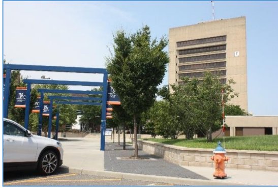
1: View looking northeast towards the NCC Student Services Center and Tower (Administration) Building from the NCC West Parking Lot.
