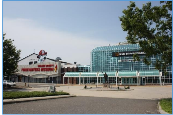
2: View looking north towards the Nassau County Firefighters Museum and Cradle of Aviation Museum within Museum Row from the eastern parking lot.
