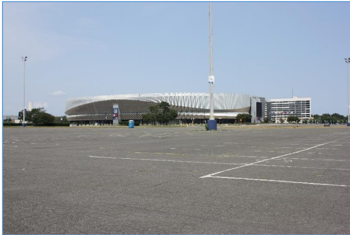
View looking northeast towards the existing Coliseum building and surface parking lot.
