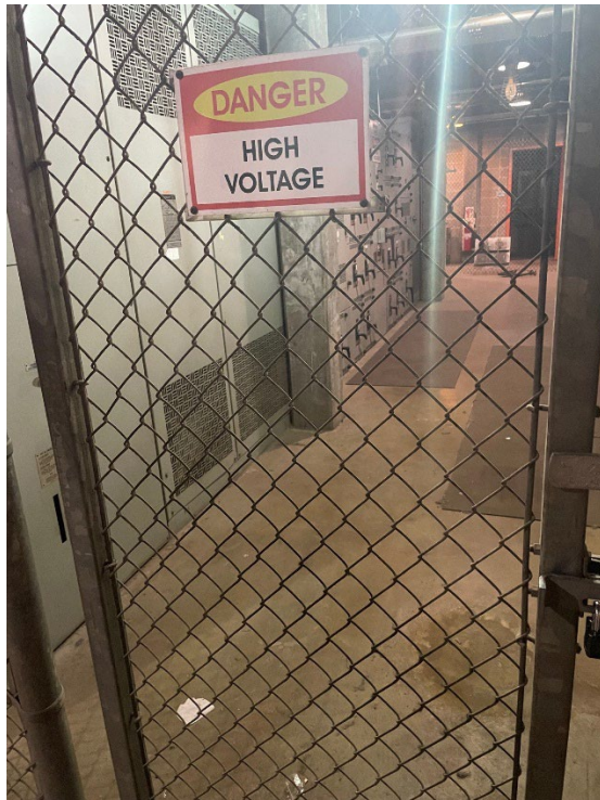
Main Switch Gear Room Assumed ACM Panels
