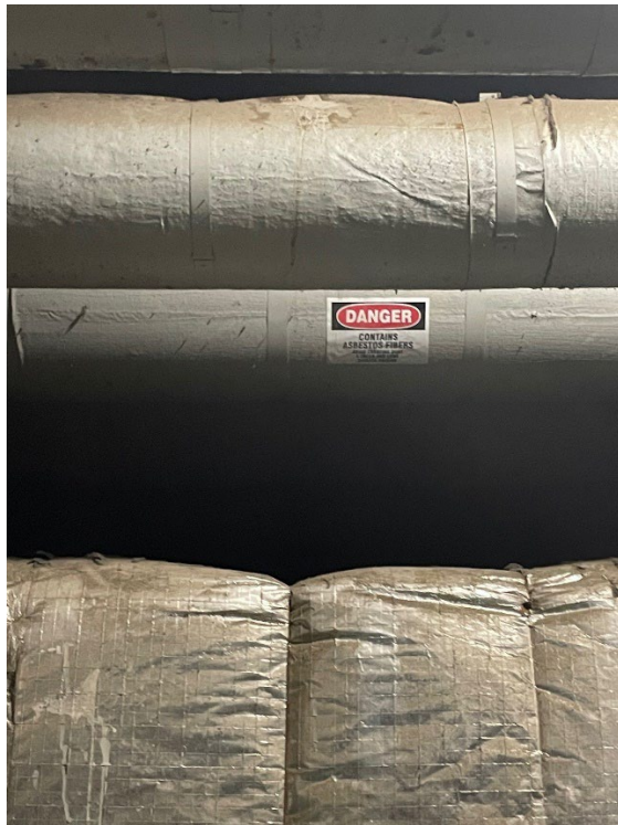
Pipe Alley Old Steam Lines ACM
