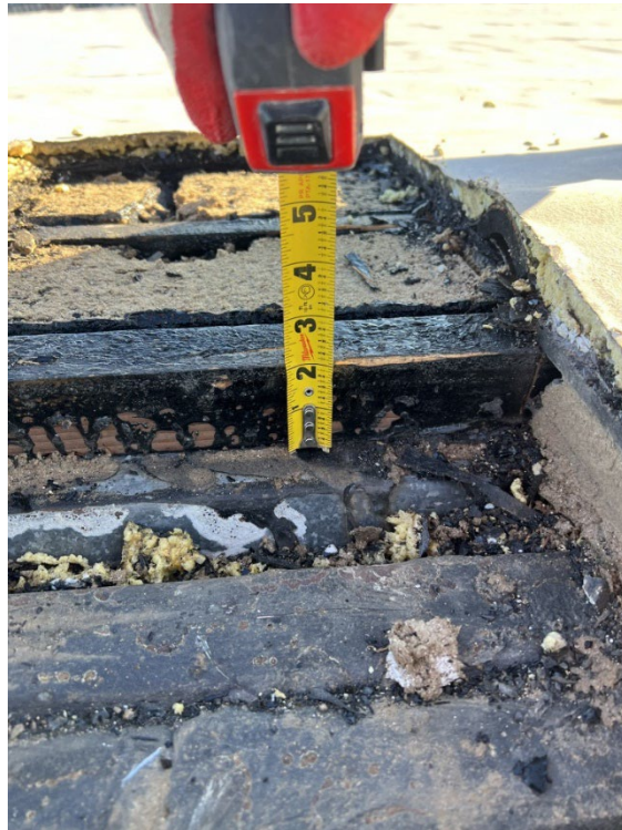
NVM Roof with ACM tar-impregnated wood strips
