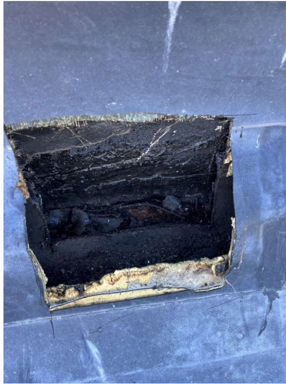
Drawing H-110 | NVM Roof Gutter Side and Base ACM Tar and Membranes | Date: 12-2023
