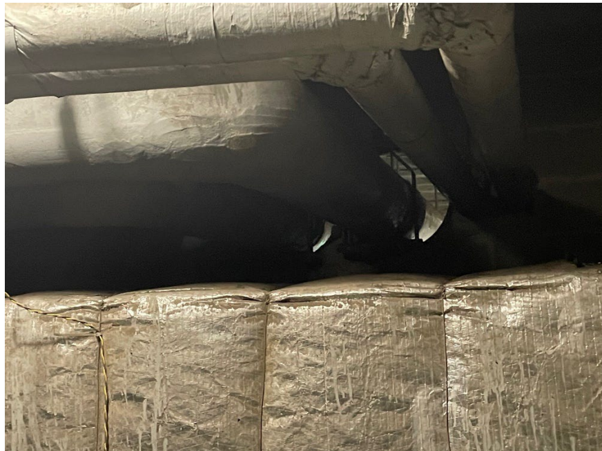
Pipe Alley Old ACM Steam Lines Turn into AC-1 and AC-2
