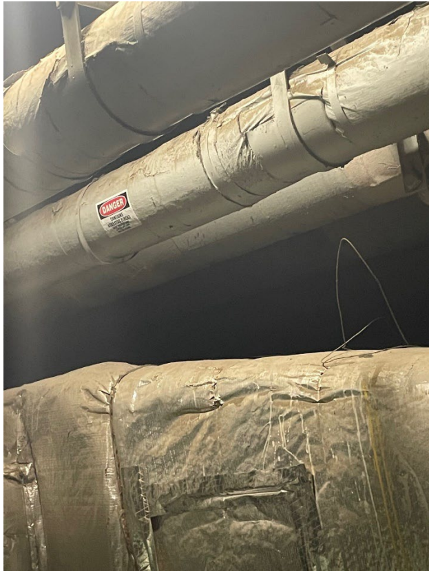
Pipe Alley Old Steam Lines ACM
