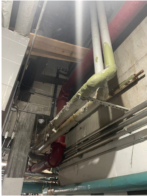
Mech Room by Engineering Office ACM Pipe and Fittings
