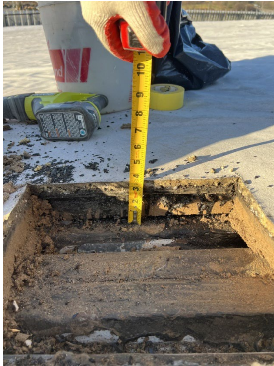
NVM Roof Multiple ACM Membranes
