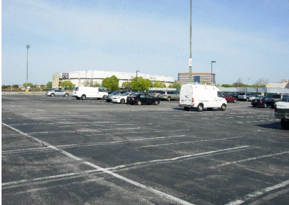
Photograph 1. Looking northwest at the Nassau Veterans Memorial Coliseum near the center of the project area.
