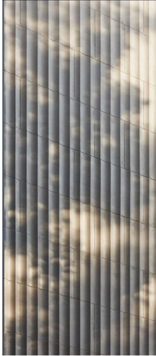
C1 - CONCRETE (Formliner)
