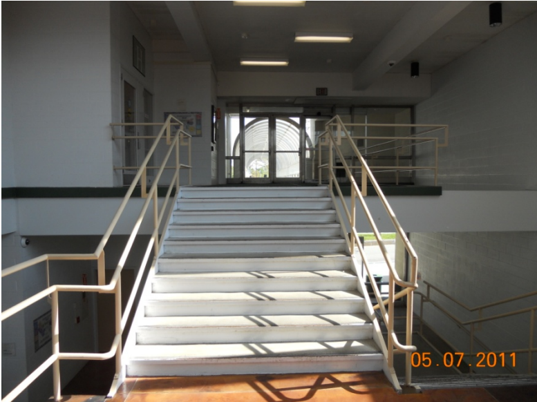
Staircase from the second floor landing to the tunnel
