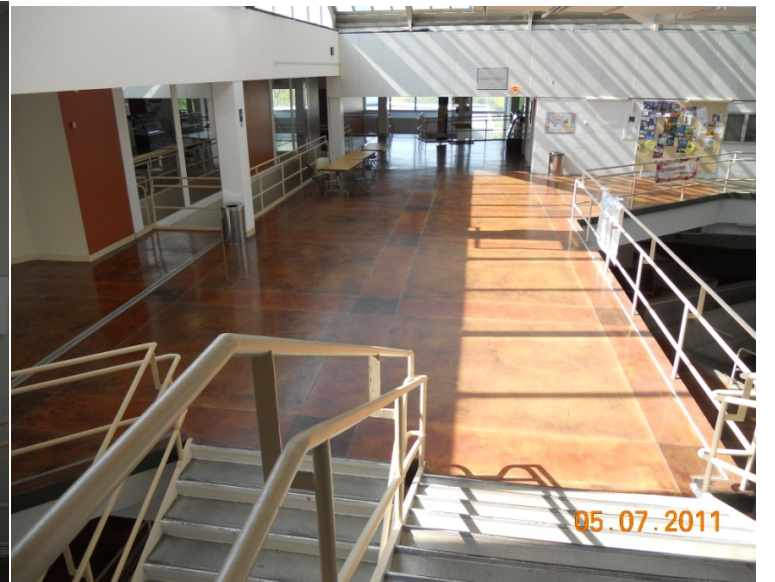
View from the tunnel to the second floor landing
