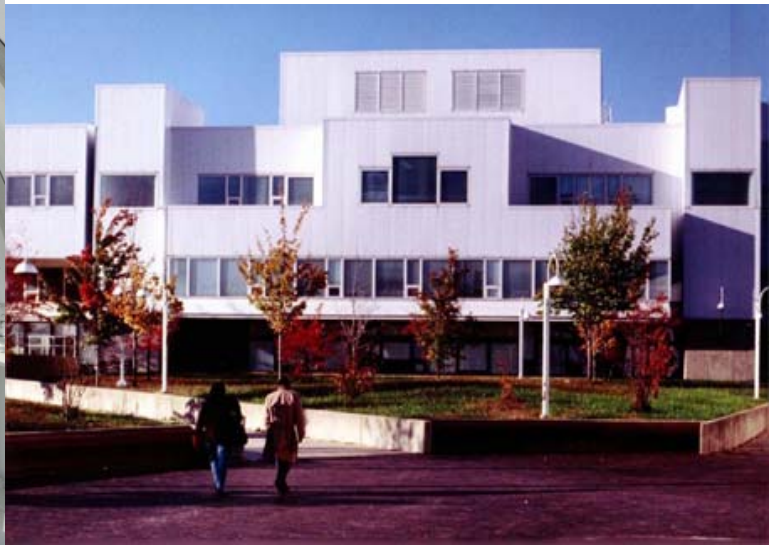
Campus Center, rear of building
