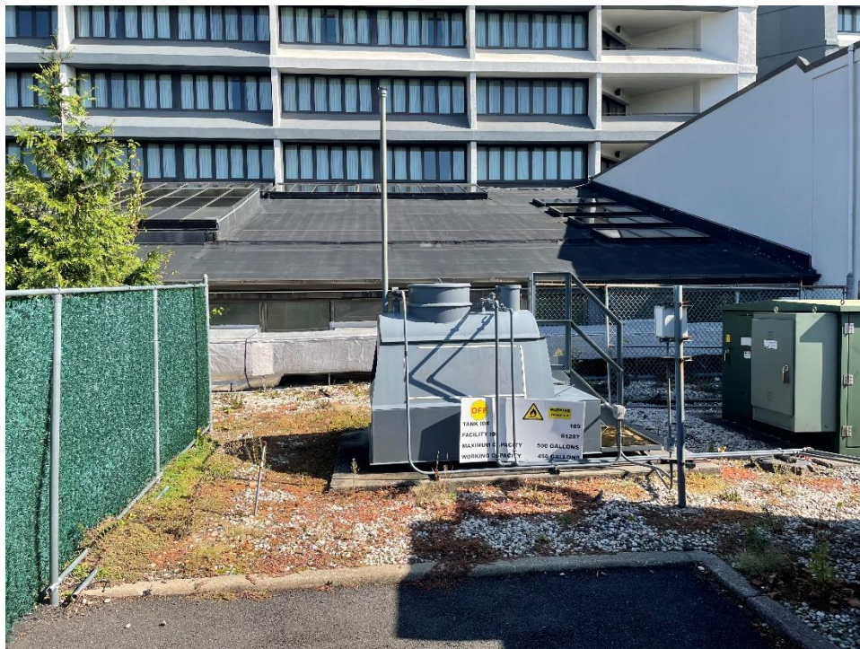
Photograph 14 – View of 500-gallon diesel fuel oil AST in the southern part of the hotel campus, facing north.
