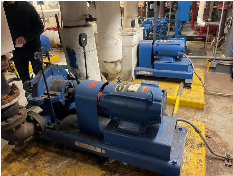
Photograph 16 – Representative view of electric elevator mechanical room, facing northwest.
