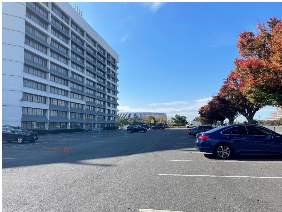
Photograph 2 – General view of the northern asphalt-paved parking area of the Subject Property, facing west.
