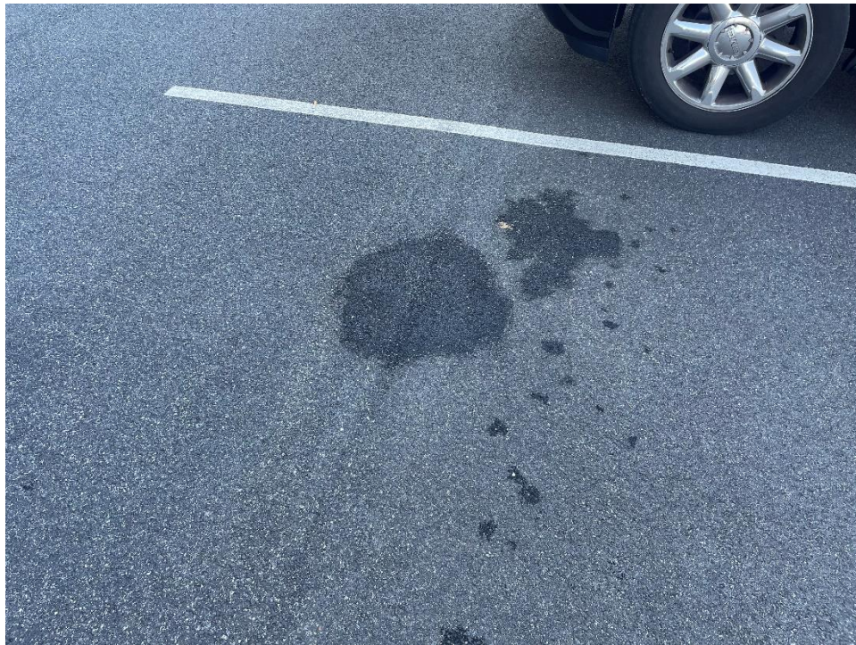
Photograph 24 – Representative view of de minimus staining throughout vehicle parking areas, facing west.
