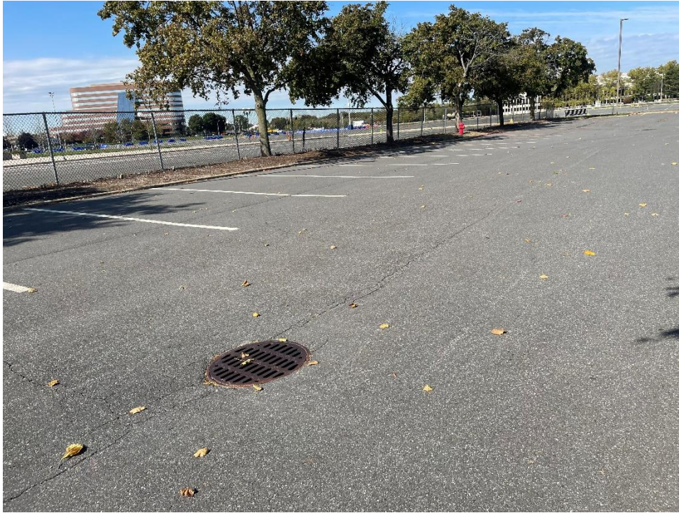
Photograph 7 – Representative view of drainage structures throughout the Subject Property, facing northwest.
