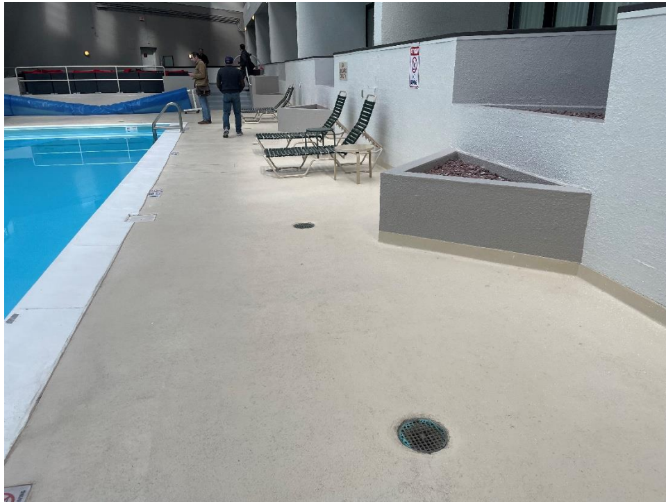
Photograph 11 – General view of floor drains throughout pool area, facing south.
