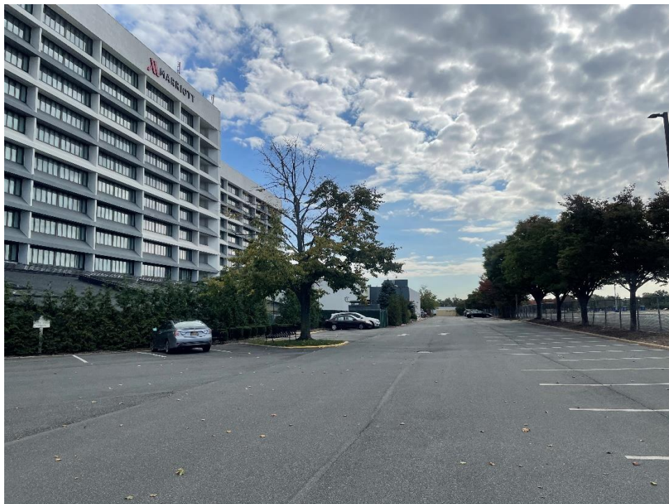
Photograph 4 – General view of asphalt-paved parking area in the western part of the Subject Property, facing south.
