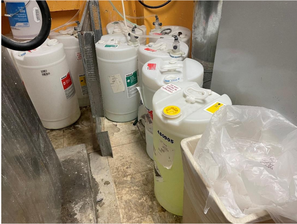
Photograph 17 – General view of laundry chemical storage area, facing west.
