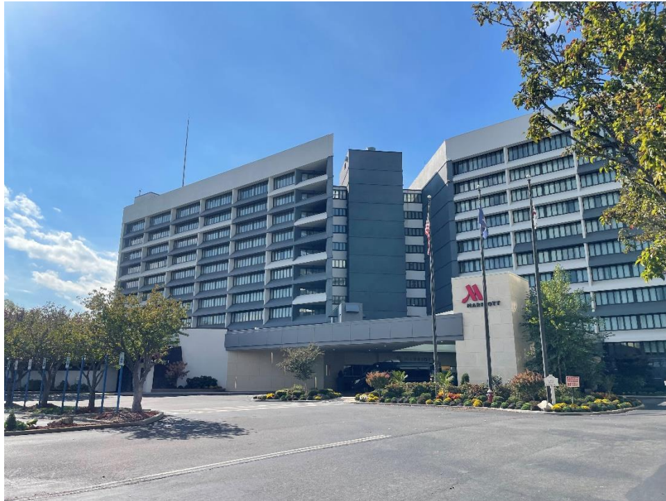
Photograph 1 – General view of the Long Island Marriott building in the northern part of the Subject Property, facing west.
