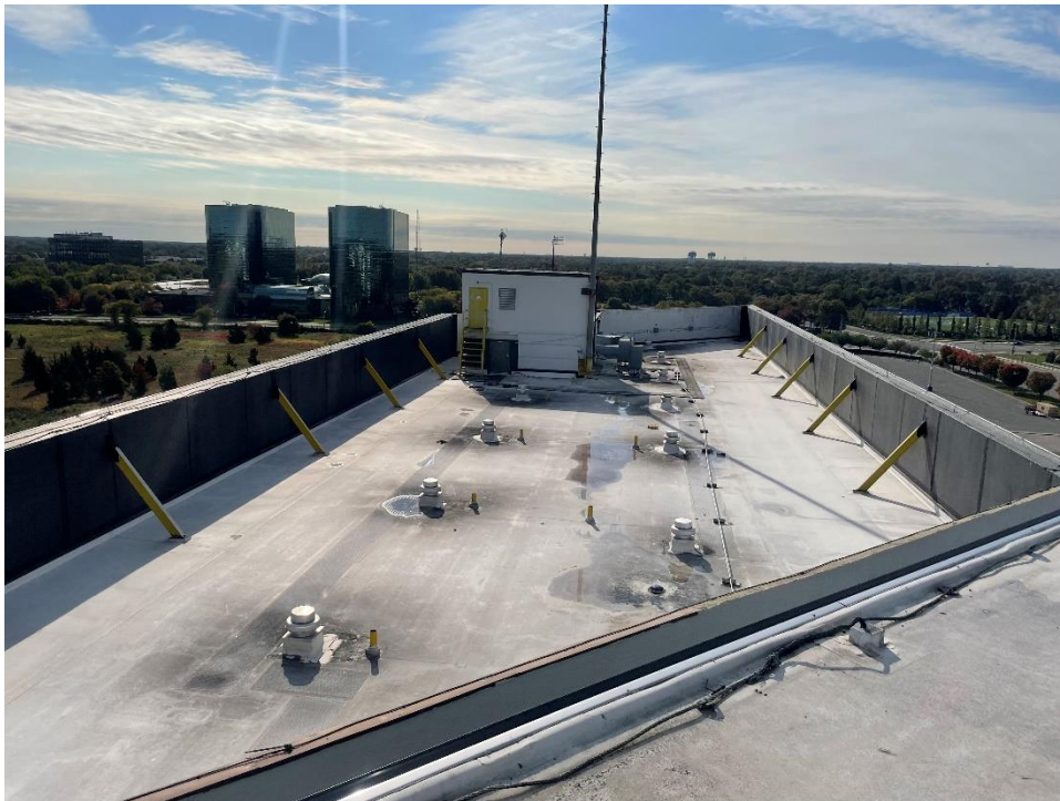
Photograph 20 – General view of building rooftop, facing south.
