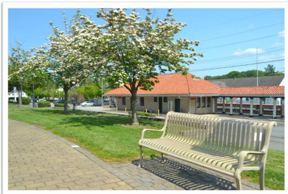
Many Nassau County residents commute to New York City and its outer boroughs for employment, cultural events and healthcare. Pictured here is the Long Island Railroad (LIRR) station in Locust Valley.
