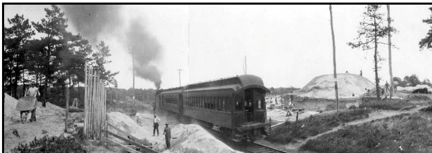
Central Ave Bethpage bridge construction, Vanderbilt Cup Races, 1908
