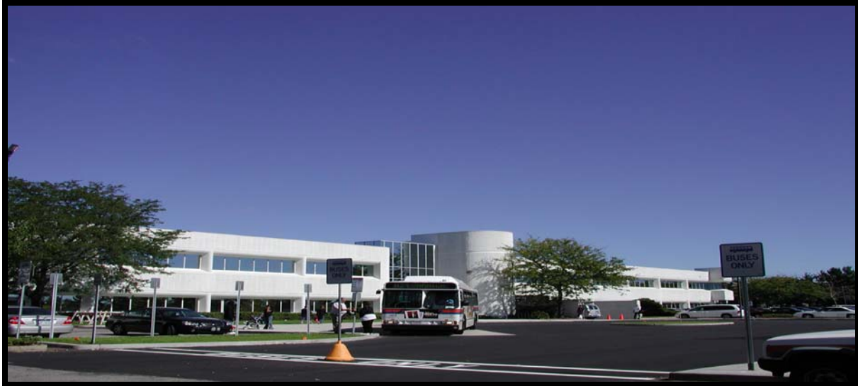
Nassau County Health and Human Services Building 60 Charles Lindbergh Blvd.
