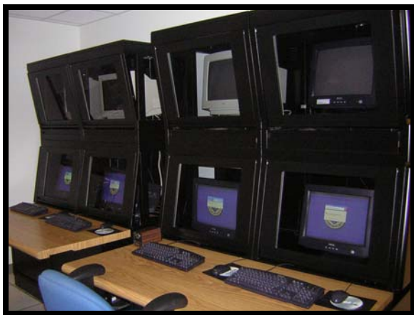
Data Center: Main Console Area
