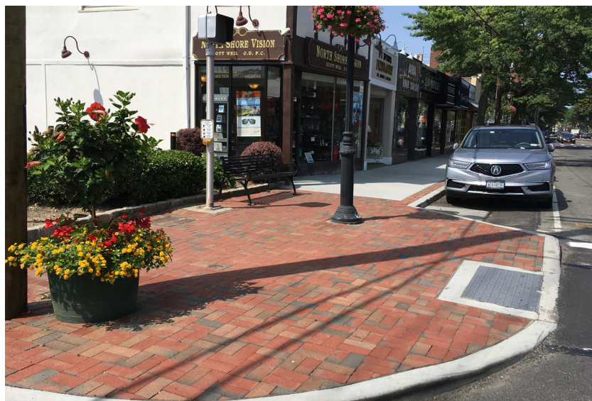
ADA Compliant brick curb extension with planters.
