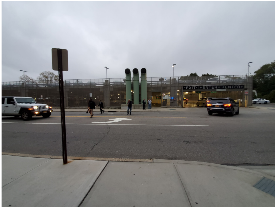
Looking south across Duffy Ave at the Town parking garage entrance.
