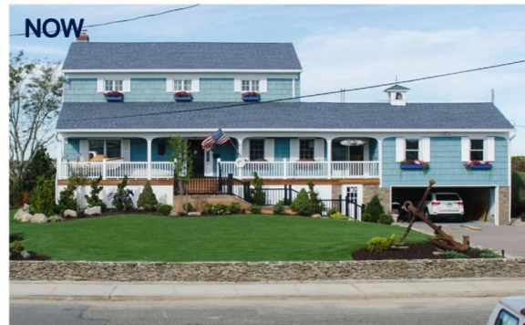
House elevation in Freeport, Long Island — Freeport, N.Y. Source: Hurricane Sandy Recovery Photos , FEMA
