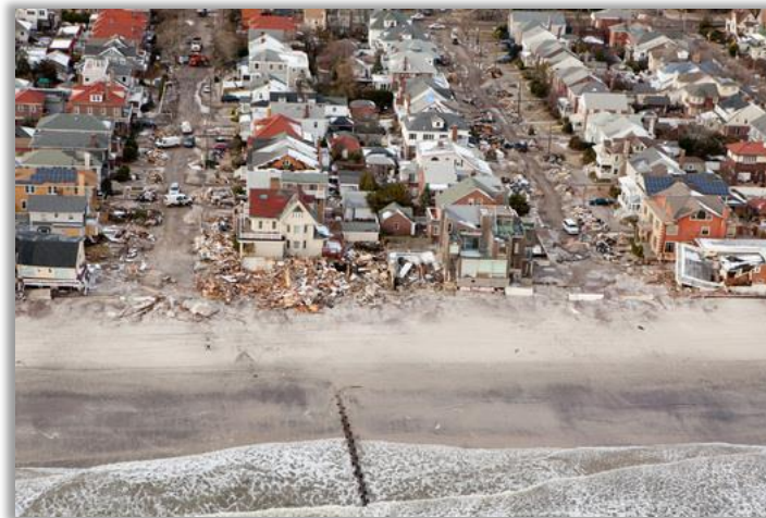
Long Beach, NY – Damage after Superstorm Sandy 2012 Source
