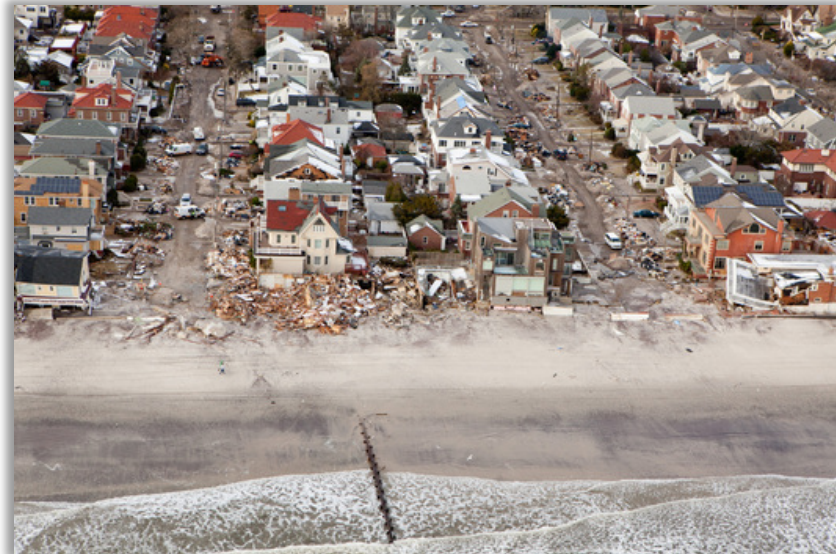
Long Beach, NY – Damage after Superstorm Sandy 2012
