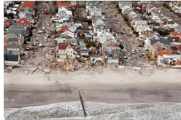
Long Beach, NY – Damage after Superstorm Sandy 2012
