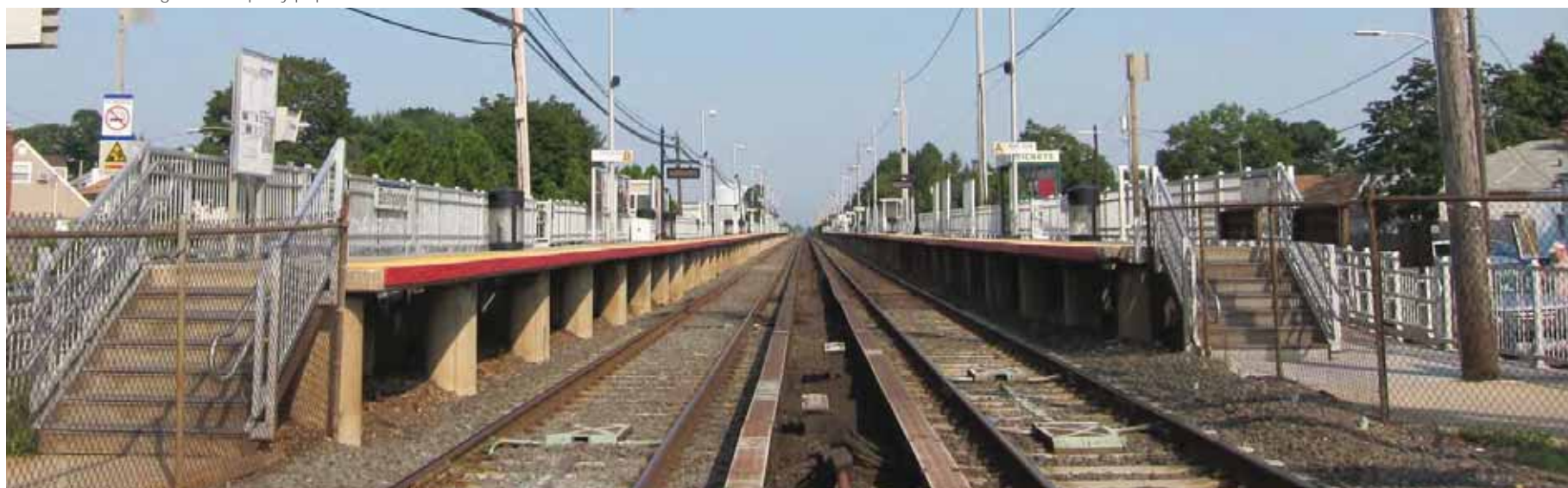
At-grade platforms at Bethpage Station.
