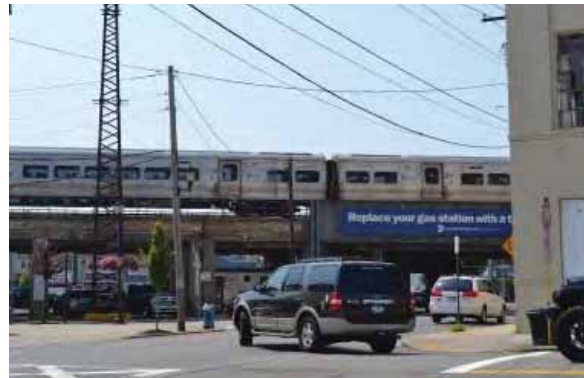
Lynbrook's "feather building" (right) presents an ideal site for mixed-use development near the station.
