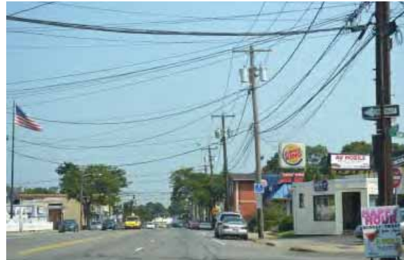
Pedestrian safety improvements are needed along Grand Avenue.
