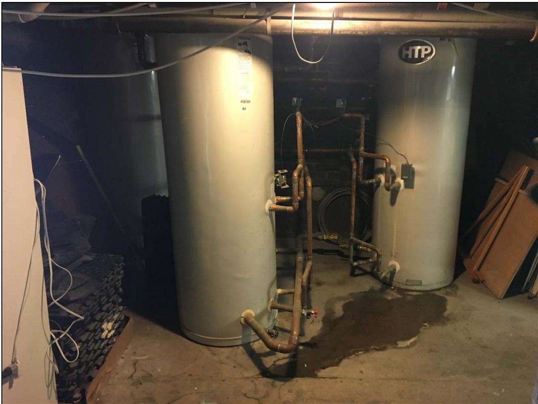
**Photograph 18: Tank with Leaking**
