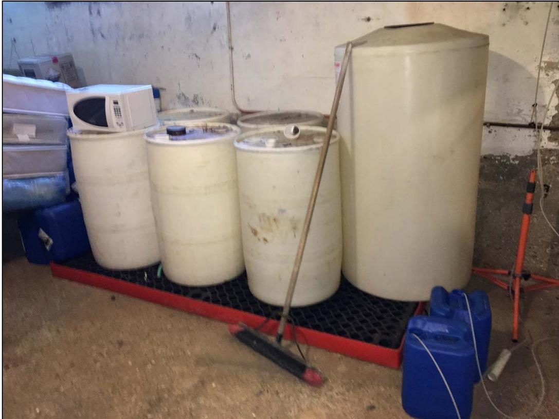
**Photograph 29: Drums Stored on Containment Pad in Pool House**
