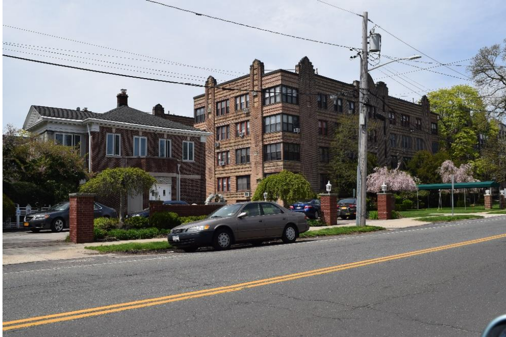
Photograph 16: View of multi-family residences on Woodmere Boulevard, northeast of the subject property.
