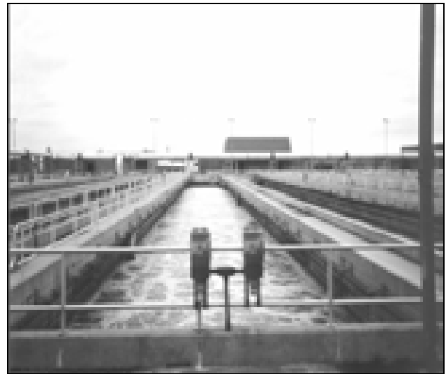
A view of Nassau County's Cedar Creek Water Pollution Control Facility.
