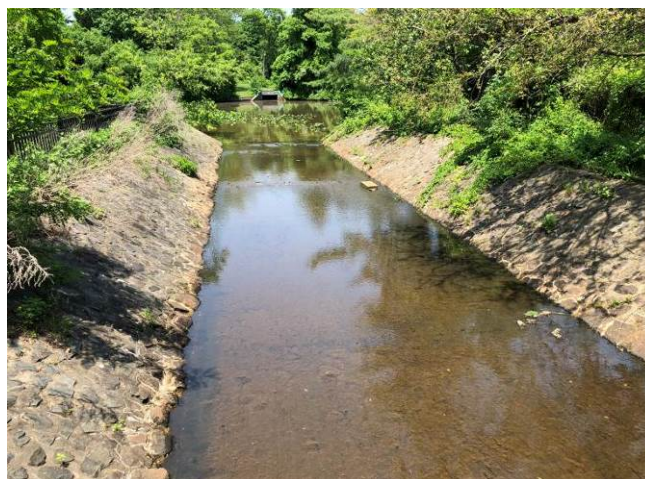
Photo 10. Photograph taken from Wateredge Avenue looking north into Caroline’s Pond. Concrete trapezoidal channel in forefront controls water surface elevations. Shallow base flow under normal conditions is not conducive for fish passage.
