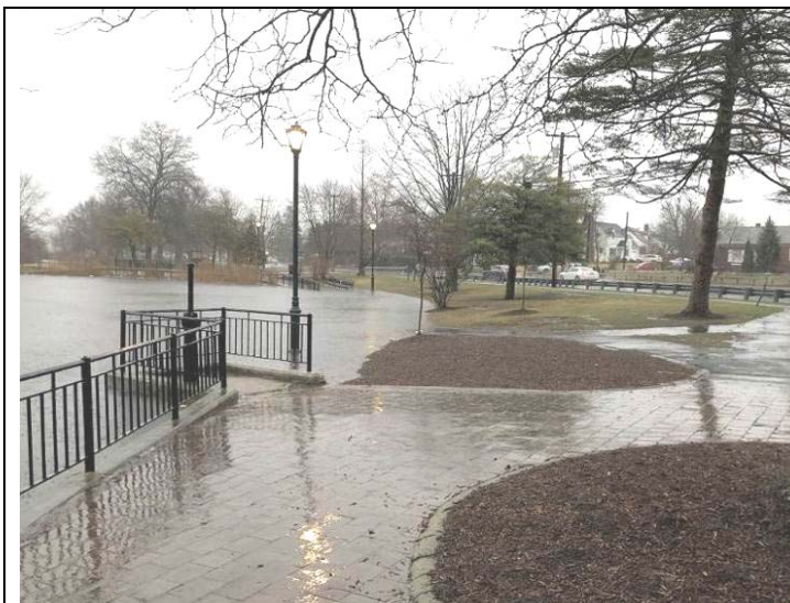
Photo 1. March 2, 2018 flooding observed in Silver Lake Park east of existing weir. Walkway is completely inundated with flood waters. Photograph taken at peak high tide.
