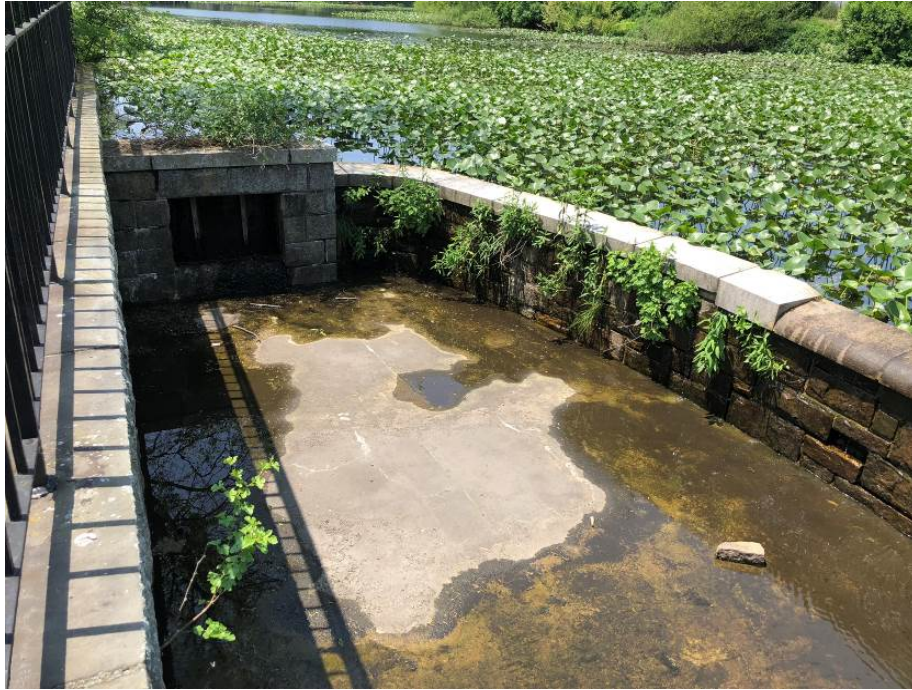
Photo 11. Weir Structure at Lofts Pond
