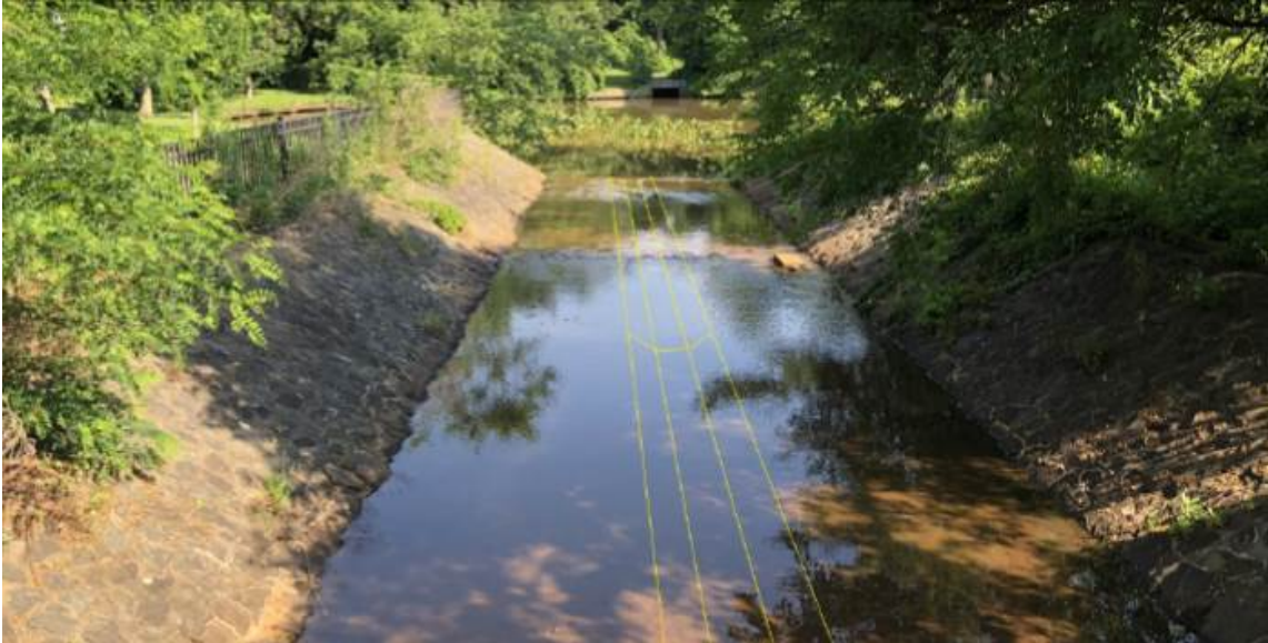
Figure IV-12. Trapezoid Channel south of Caroline’s Pond Currently Restricting Fish Passage. Proposed Location of Low Flow Channel for Fish Passage Depicted
