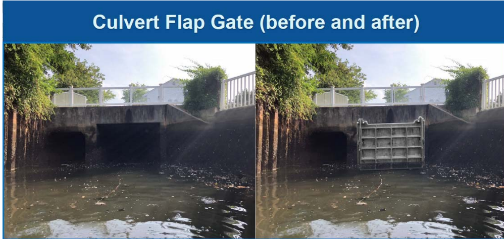
Figure IV-9. Tide Gate Photo-Simulation at Parsonage Canal Outfall
