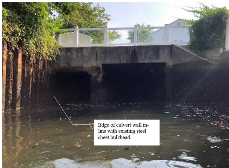
Photo 7. Photograph of existing box culvert outfalls at Parsonage Creek Canal.
