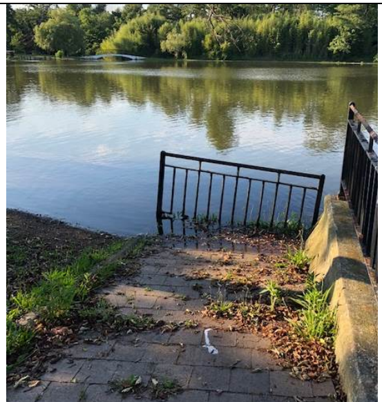
Photo 6. July 10, 2018 at Silver Lake Park west of existing weir. Tidal surge has breached the top of the existing bulkhead wall (top of wall = 3.0' NAVD)
