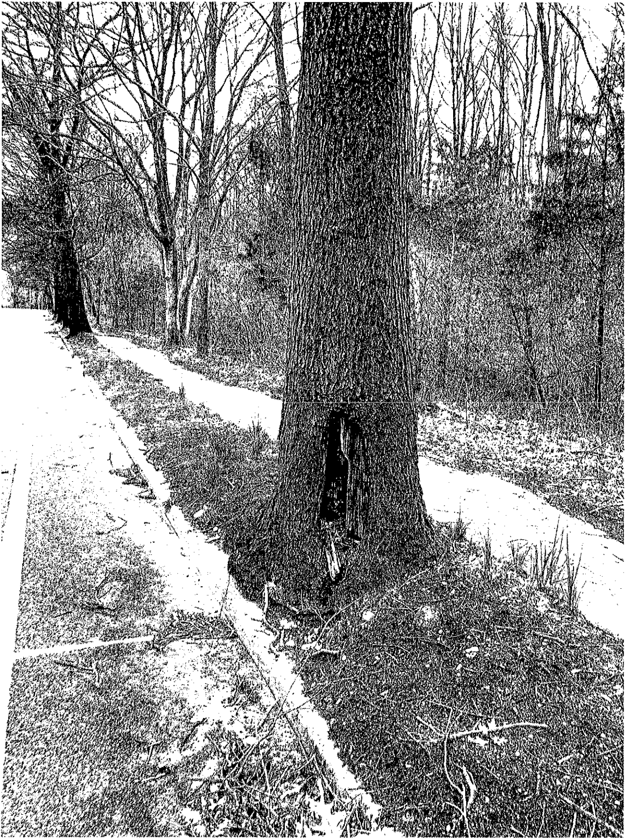
Woodbury Road Tree Removals - Example #3: Tree exhibits extensive vehicular damage and internal decay compromising its structural stability.
