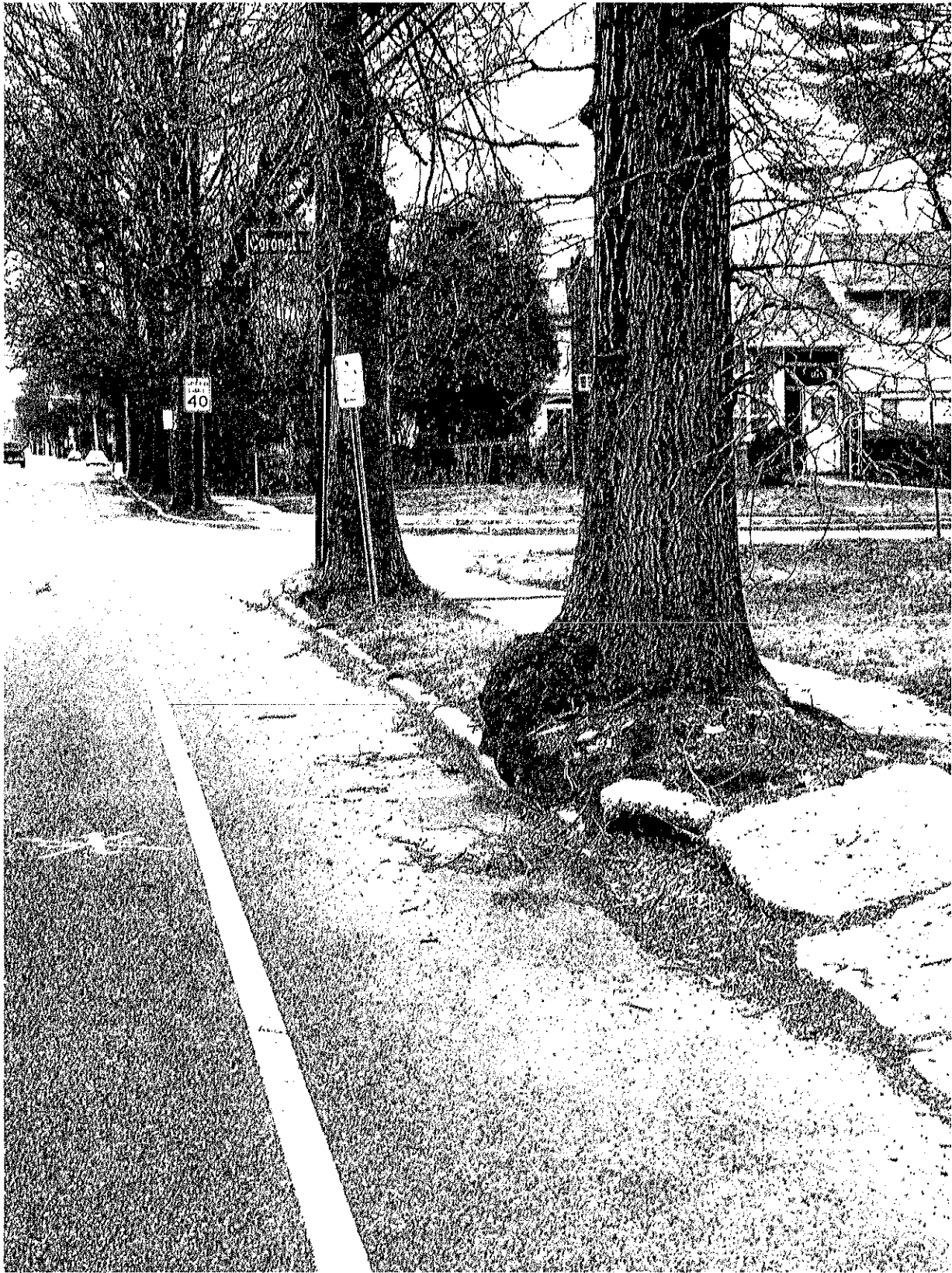
Woodbury Road Tree Removals – Example #6: Root flare far exceeds curb limits and interferes with milling.
