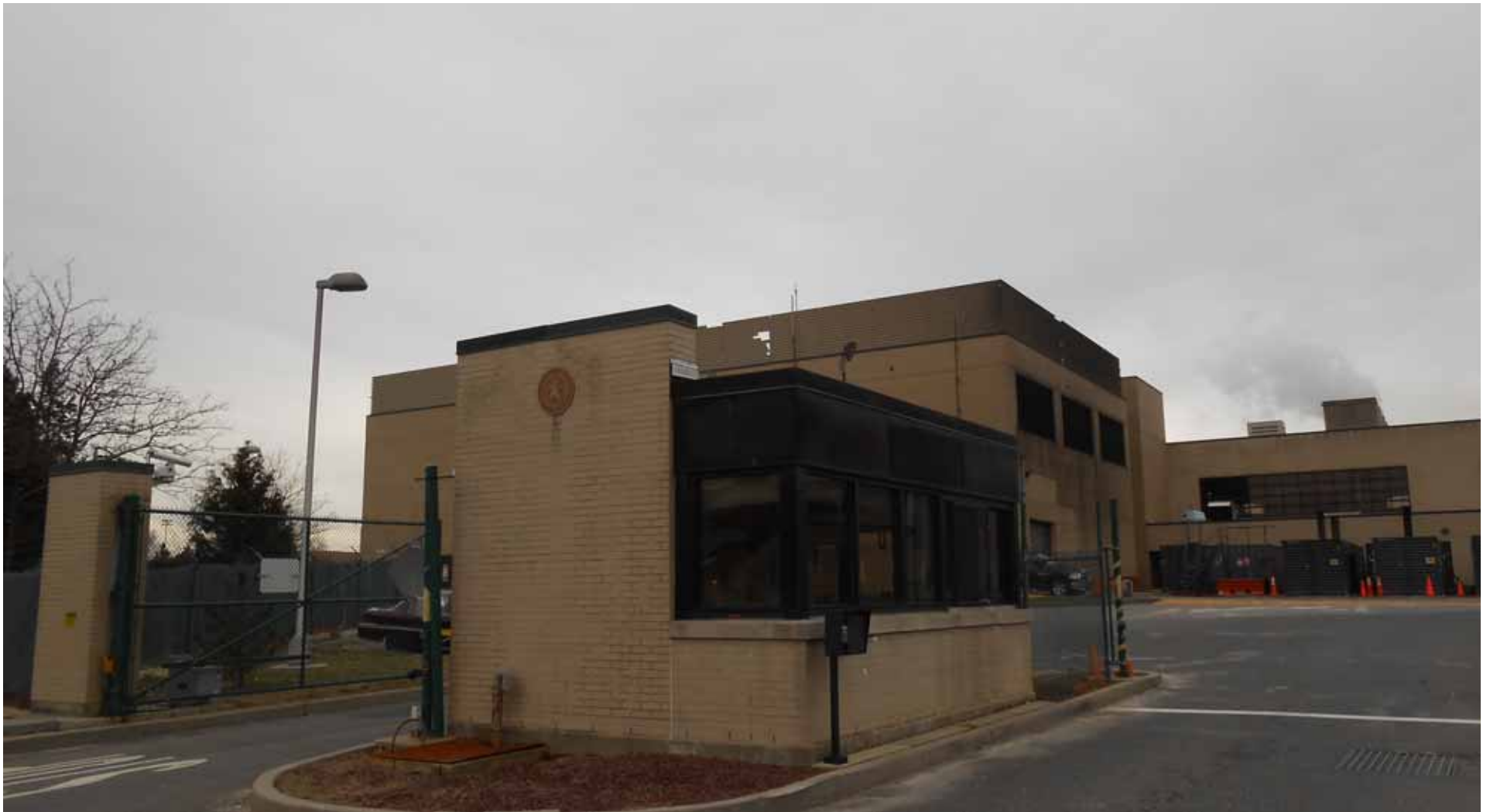
FIGURE C5 EXISTING CONDITIONS: North Gate and Guard House
