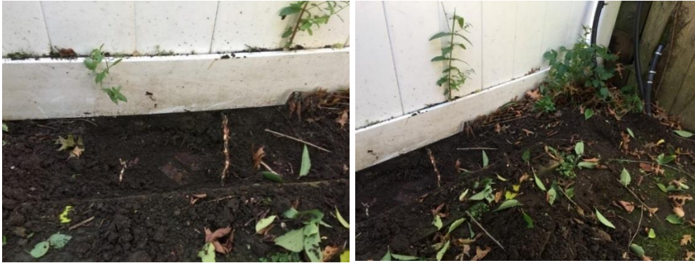
Note buried manhole under existing decorative vinyl fence
