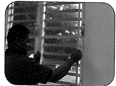
Install or repair window & door screens.
