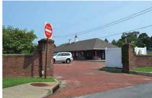
Any infill within Nassau Boulevard’s station area would need to be small in scale.
