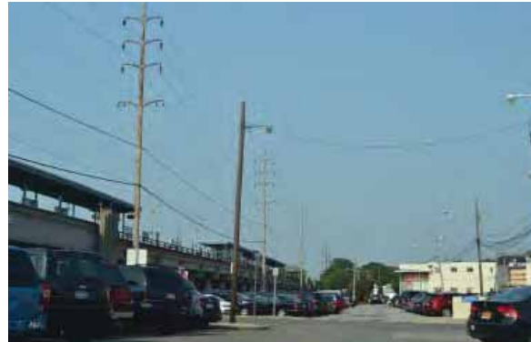
Pedestrian safety is a serious concern within Wantagh's station area.
