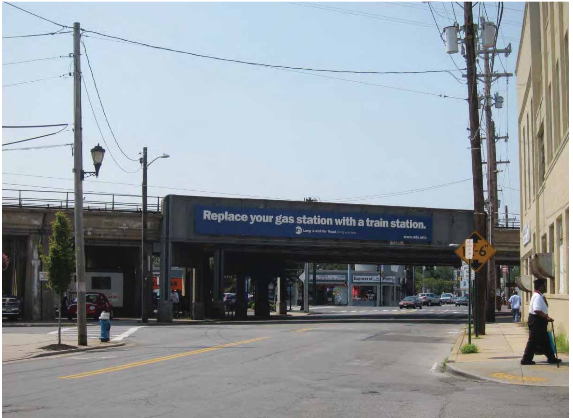
A LIRR billboard near the "Feather Building" in Lynbrook touts the benefits of taking the train instead of driving.
