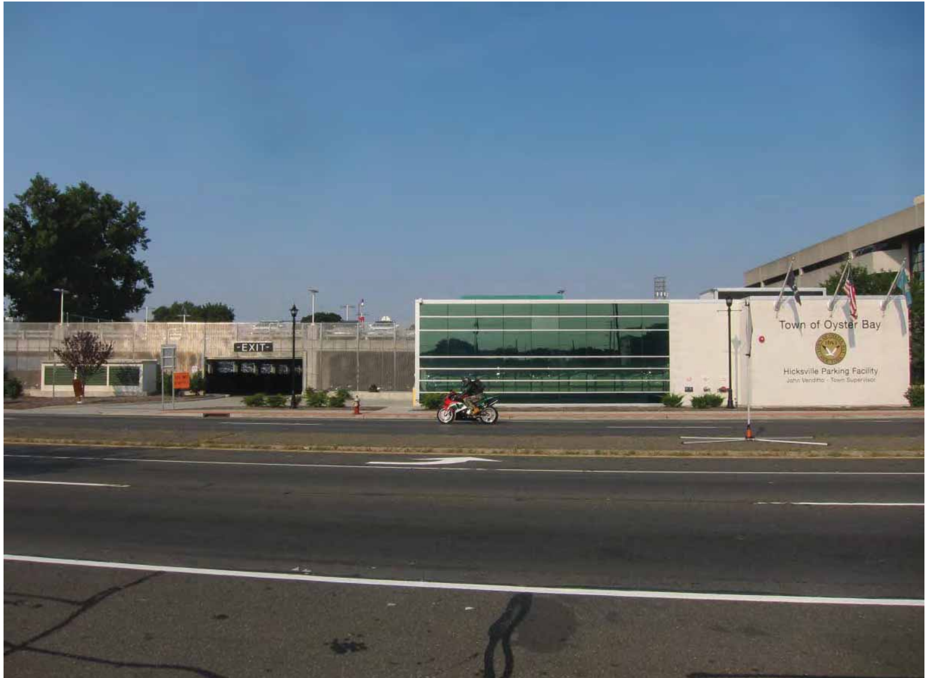
The recently completed structured parking facility at Hicksville Station.
