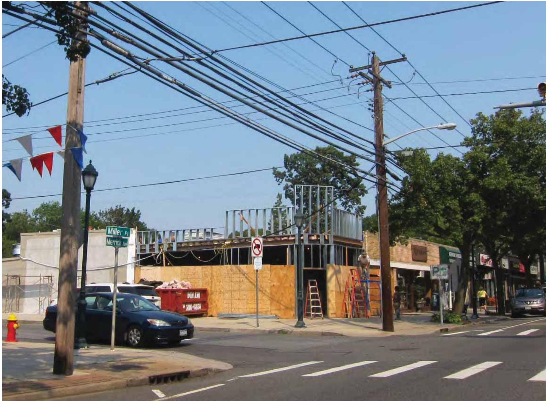
A new neighborhood-scaled development being built just north of Merrick station.
