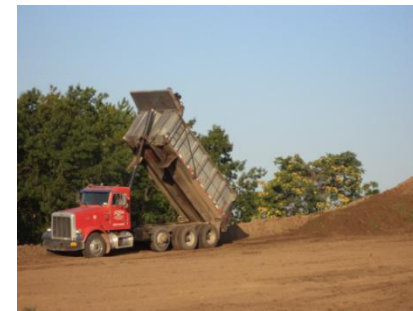
Perimeter Flood Protection – stockpile of top soil
