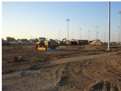
Perimeter Flood Protection – East Park Reconstruction
