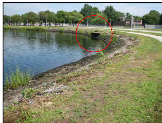
North Woodmere Waterfront and Storm Drain
