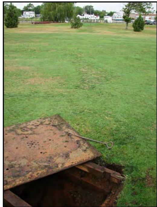
Bay Park Storm Drain
