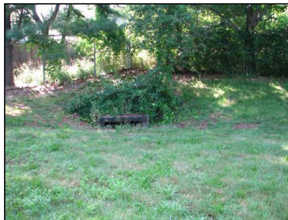
Cantiague Storm Drain
