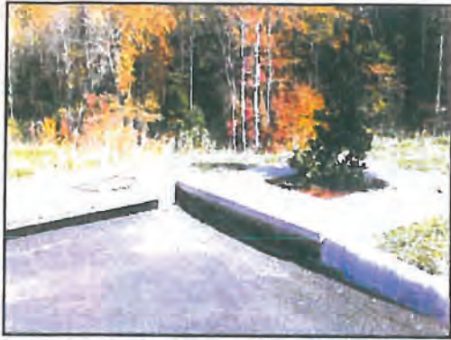
1. Inspection of Filterra and surrounding area
