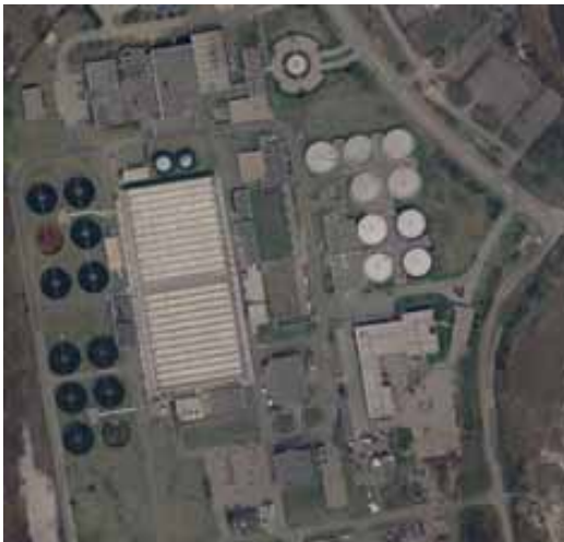
Caption: Cedar Creek Water Pollution Control Plant
