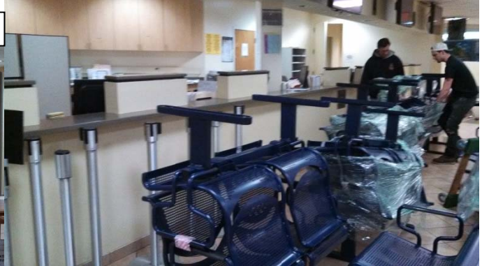
Workers start unpacking and installing the new seats.
