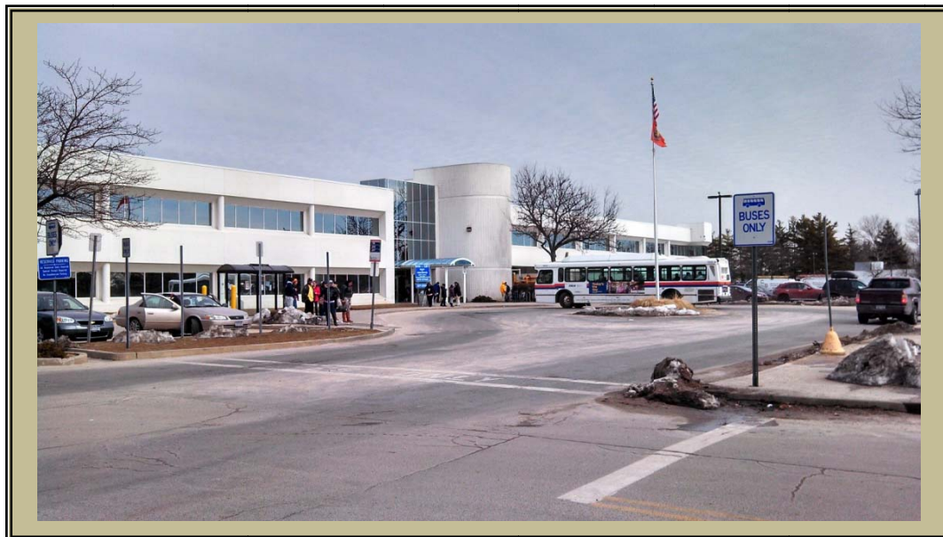
Main office complex for DSS at 60 Charles Lindbergh Blvd., Uniondale, NY
