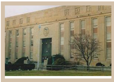
County Court House 262 Old Country Rd, Mineola
