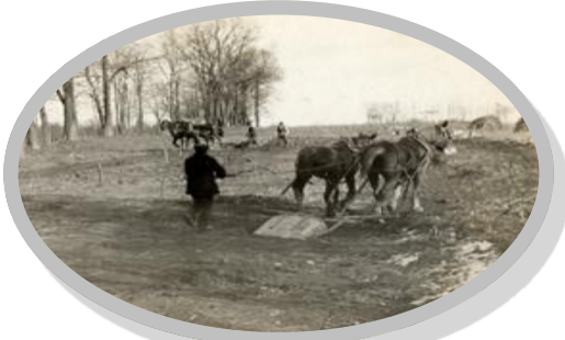
Roads being cleared on the North Shore
