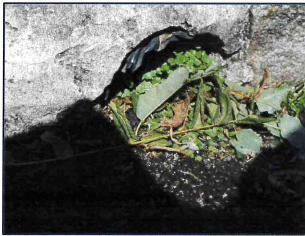
Photo of Parcel ID # 282400224630 on 8/5/2020
